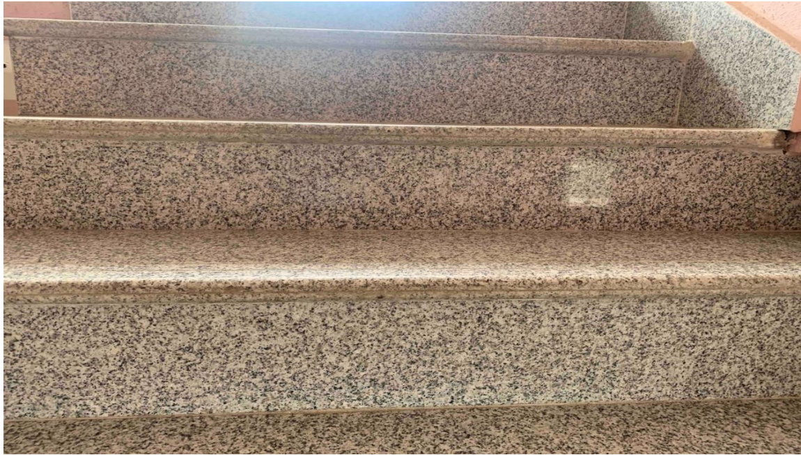
Granite laying at Staircase
